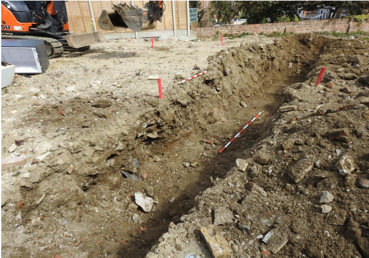
Plate 3: Showing evaluation Trench 1. Looking north, one- and two-metre scales.
